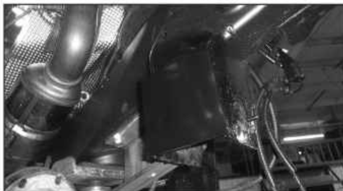
FIGURE 23 - SHOWN ALREADY PAINTED
